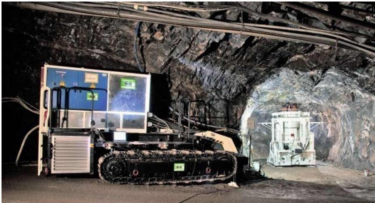
Figure C26: Boxhole borer transport unit and boring unit underground
