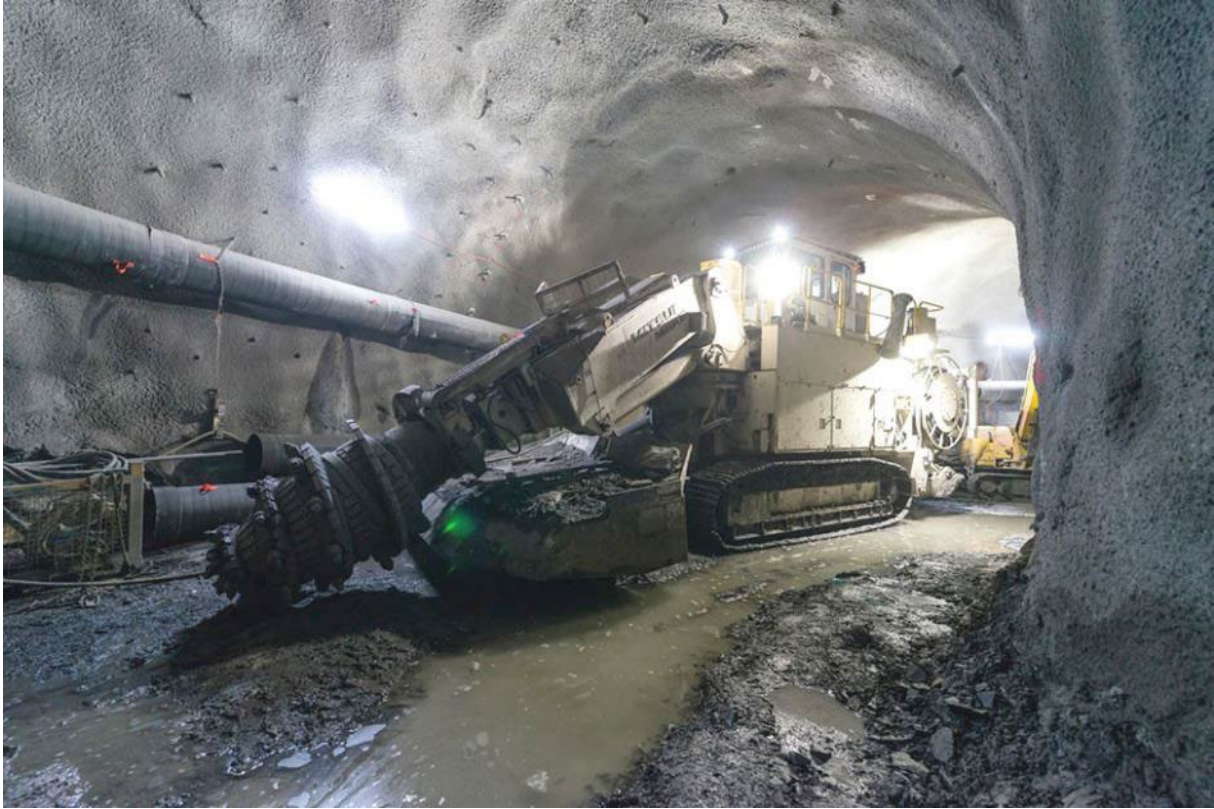
Figure C23: Roadheader tunnelling machine (sprayed concrete lined tunnel)
