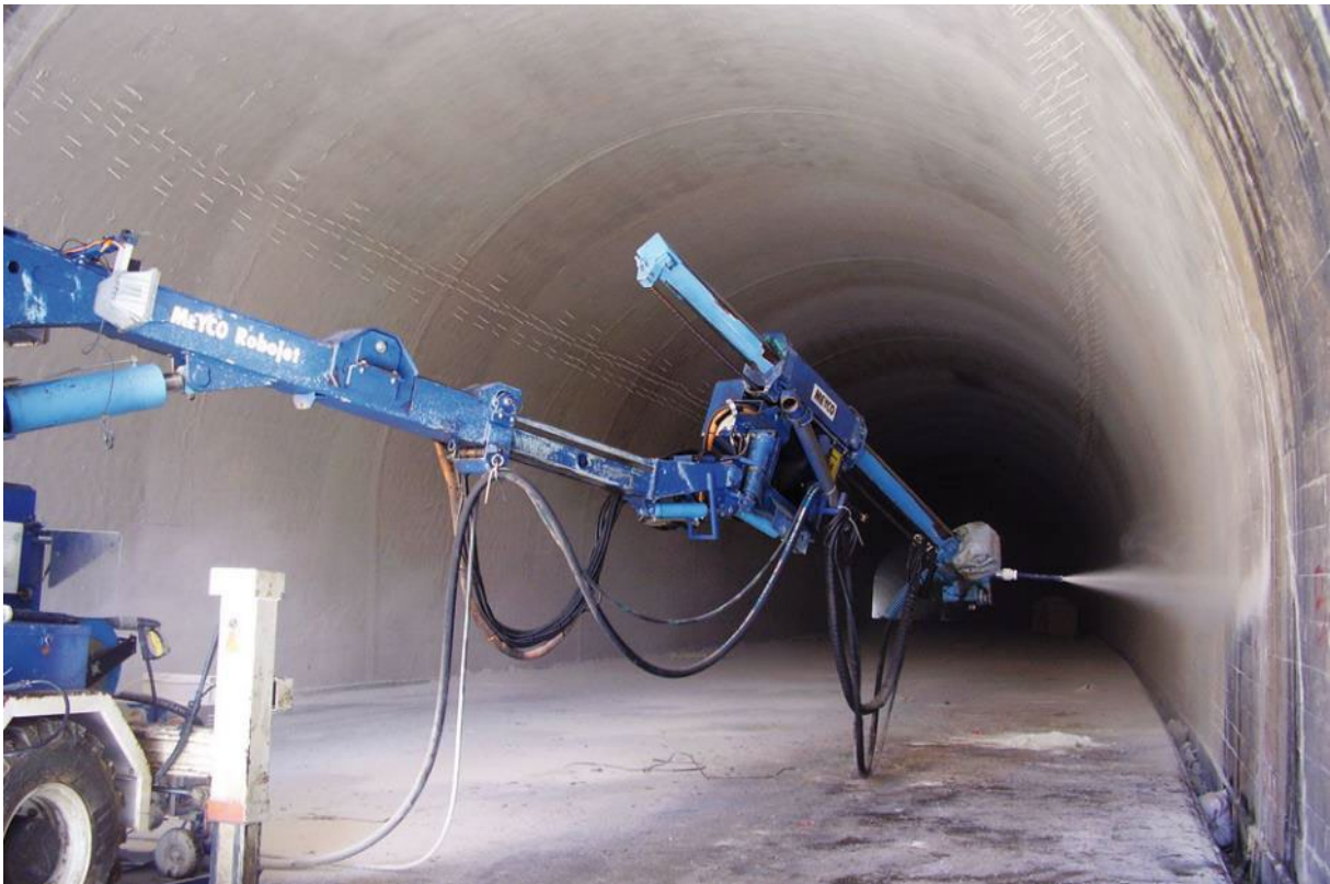
Figure C20: Robotic boom shotcrete spray machine
