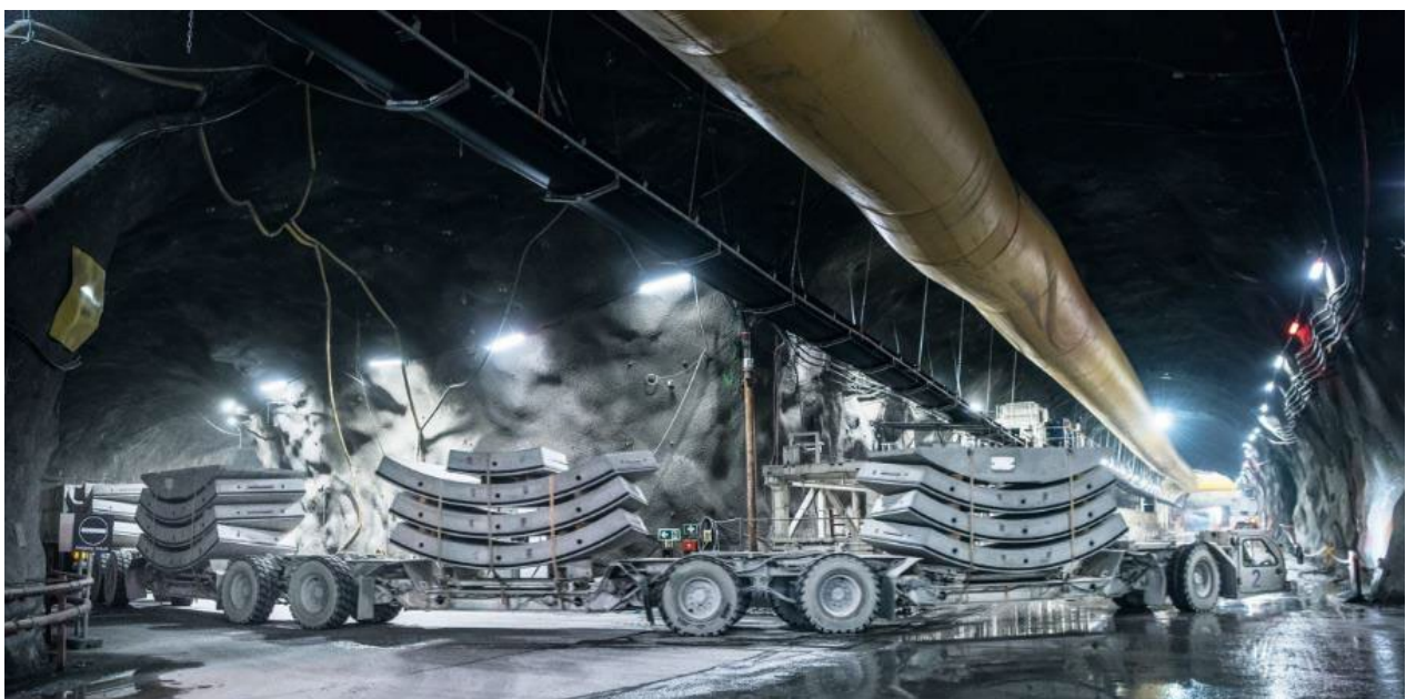
Figure C16: MSV transporting segments to TBM underground
