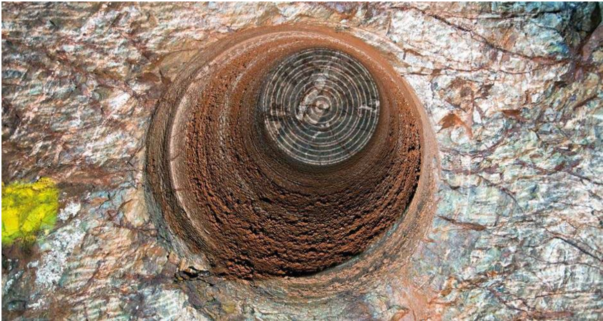
Figure C28: Example of blind drilled 'shaft'
