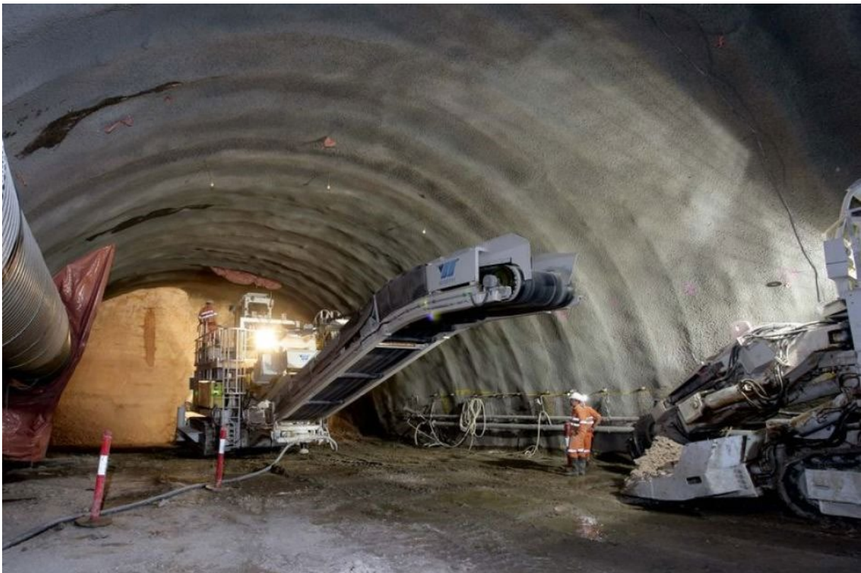
Figure C24: Roadheader tunnelling machines (sprayed concrete lined tunnel)
