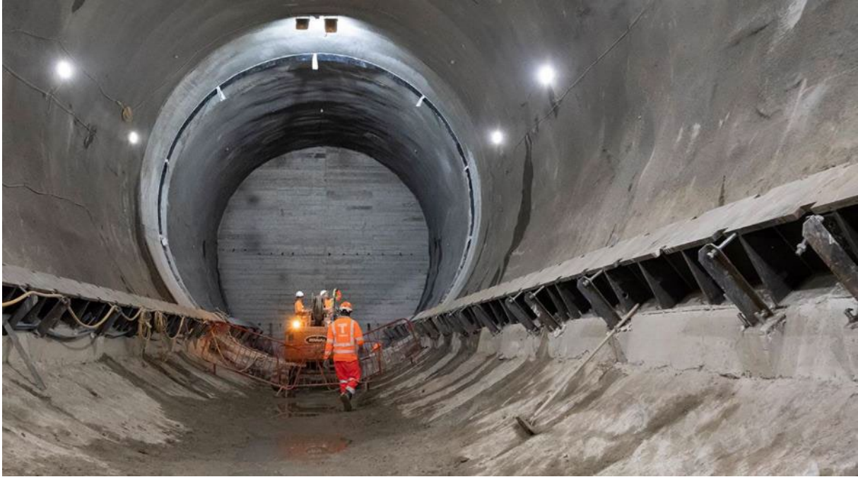
Figure C17: Underground TBM assembly chamber (© Thames Tideway)
