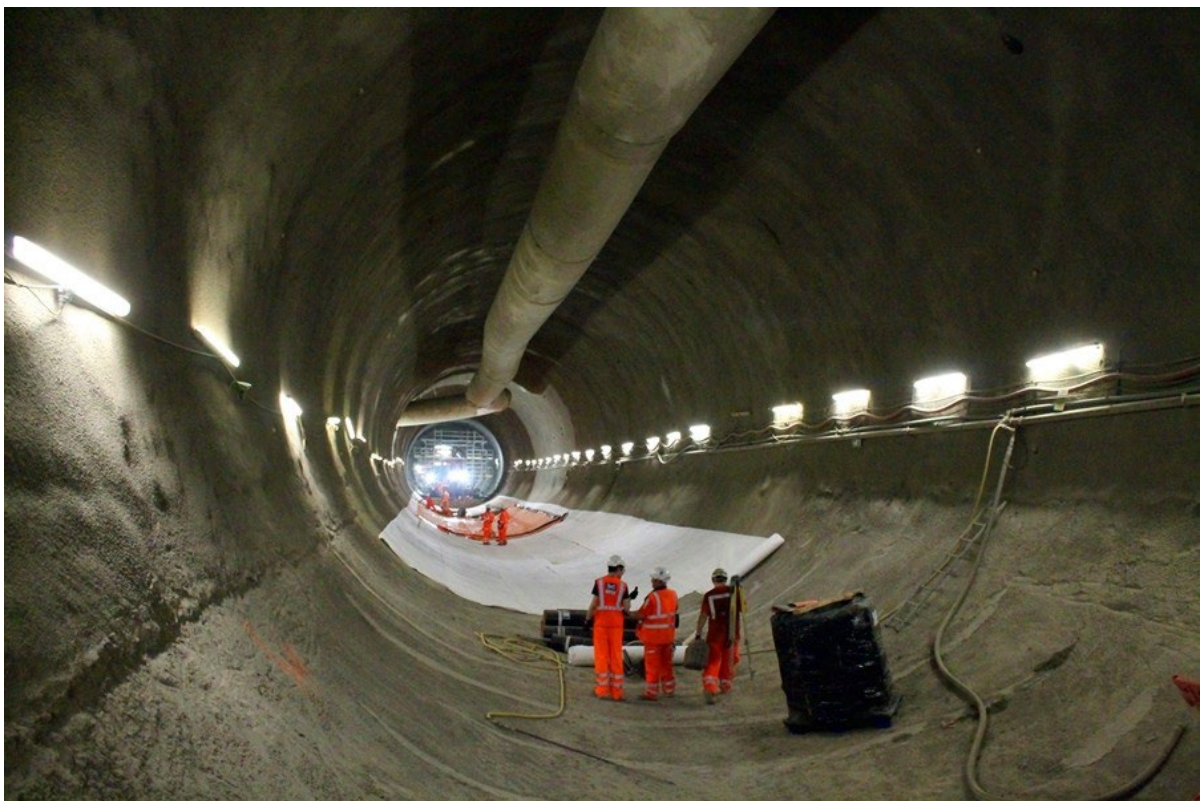
Figure C22: 12m diameter SCL tunnel (© Crossrail Ltd)
