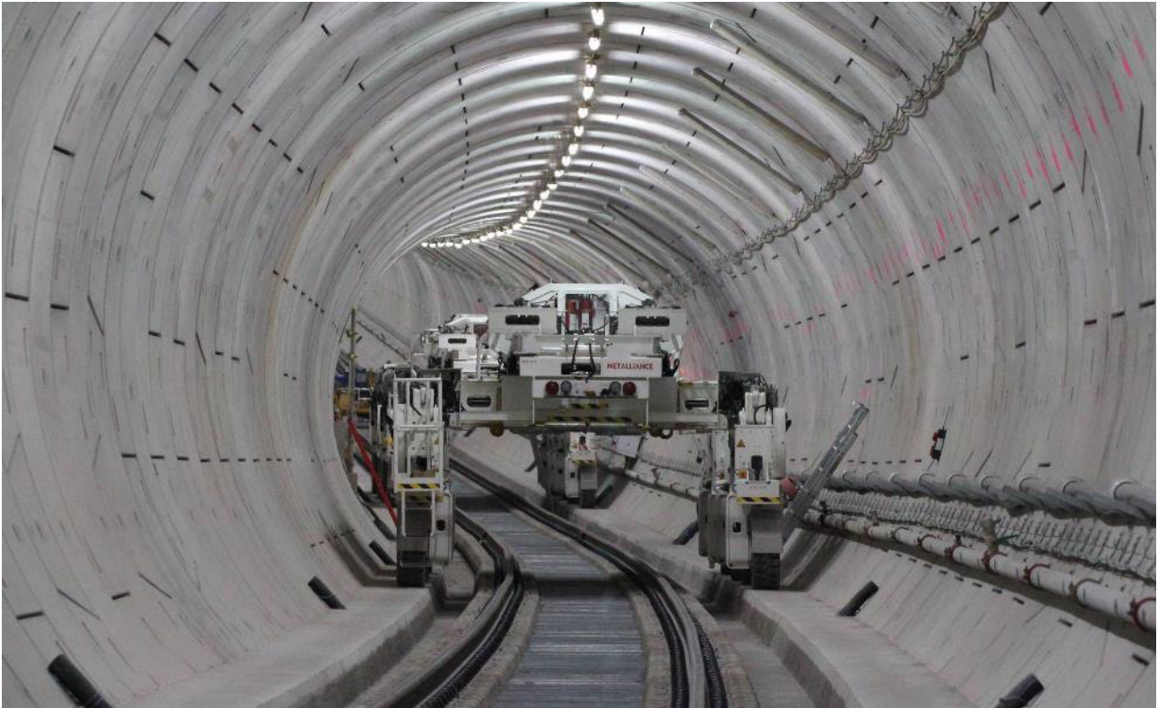
Figure C10: Multi-purpose gantry used for tunnel fit-out (© Crossrail Ltd)
