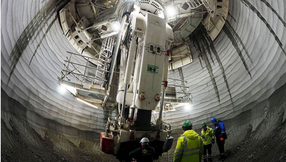
Figure C2: SBR during sinking in frozen ground (© Herrenknecht)
