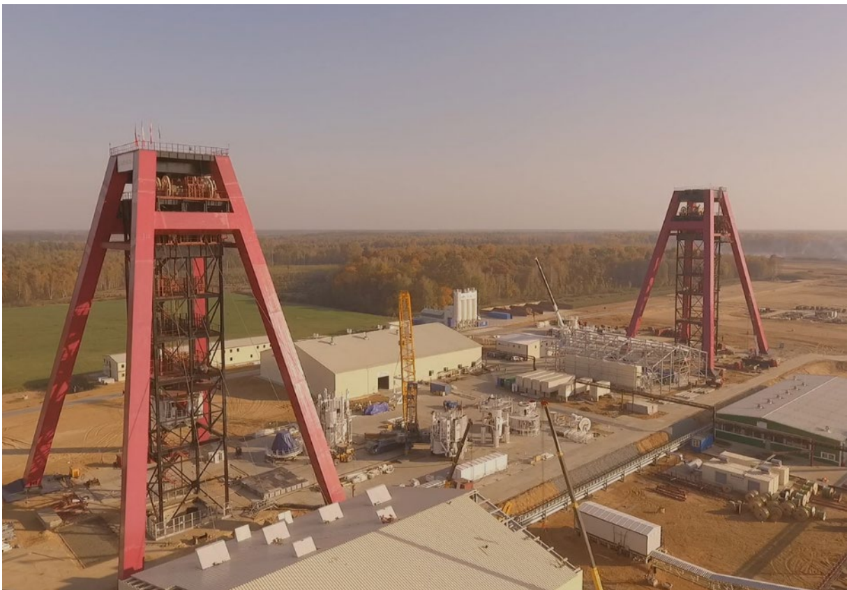
Figure C3: Typical modern shaft sinking headframes and winder houses
