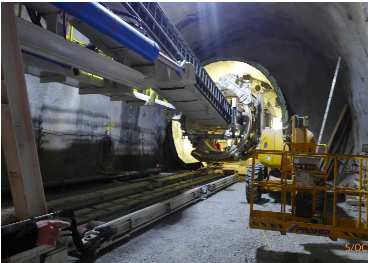
Figure C18: TBM erection within a SCL assembly chamber
