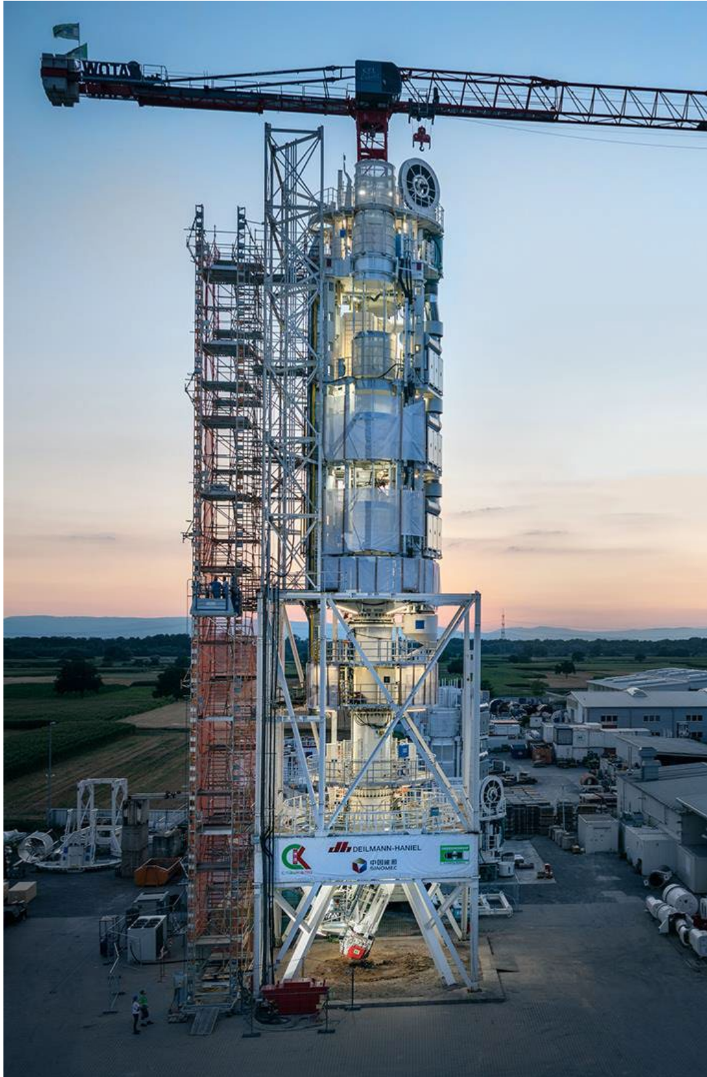
Figure C1: SBR assembled on surface (© Herrenknecht)
