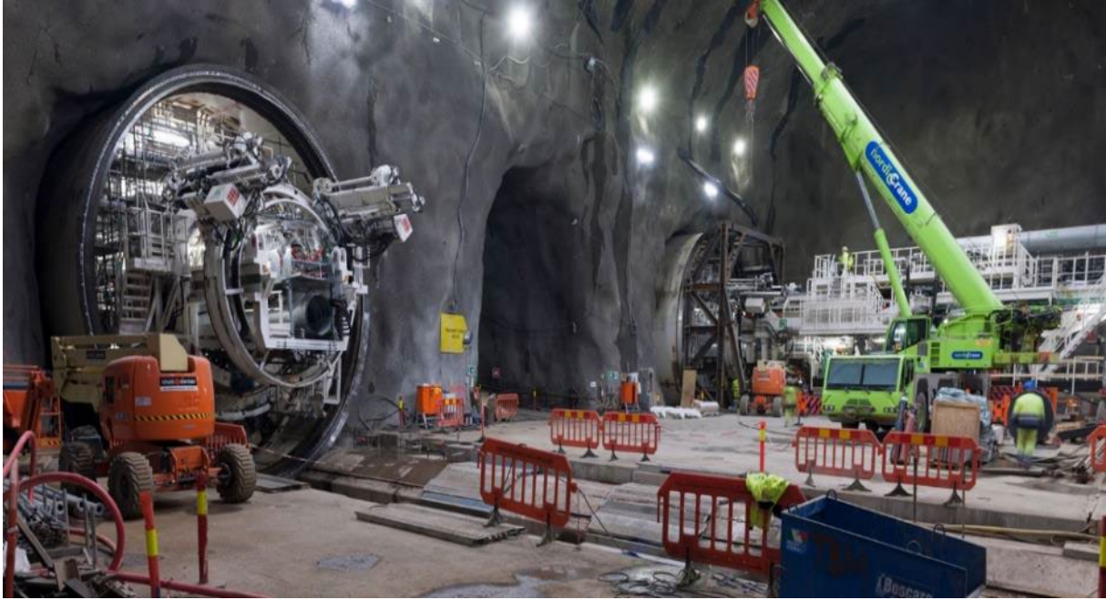
Figure C19: Underground TBM assembly chamber
