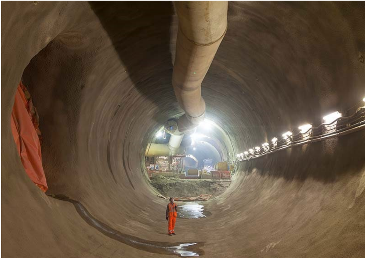
Figure C21: 12m diameter SCL tunnel (© Crossrail Ltd)
